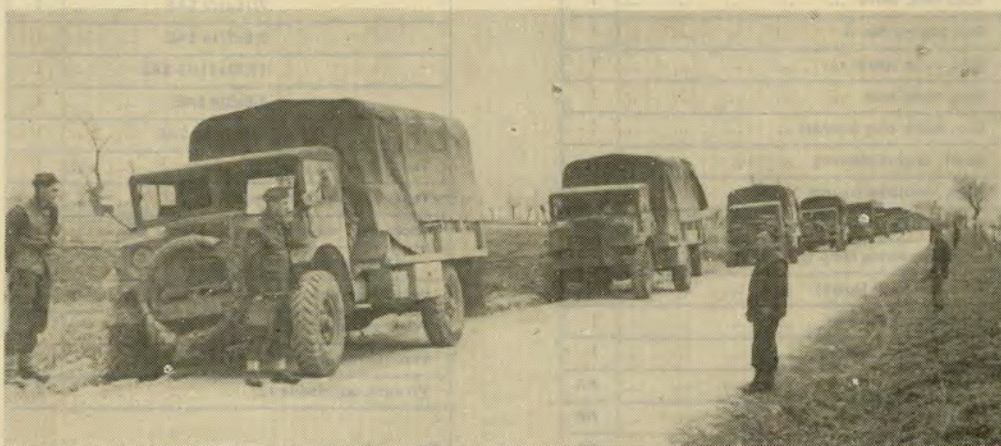
Above photograph shows a convoy halted, with vehicles in "closed-up" spacing, along right hand verge. This in line with the "Drive-on-the-right" rule of the road, now used by the armies on the continent, and promulgated in 21 Army Group orders. In accordance with standing orders, co-drivers are out across the road ready to pass orders or regulate other traffic.
