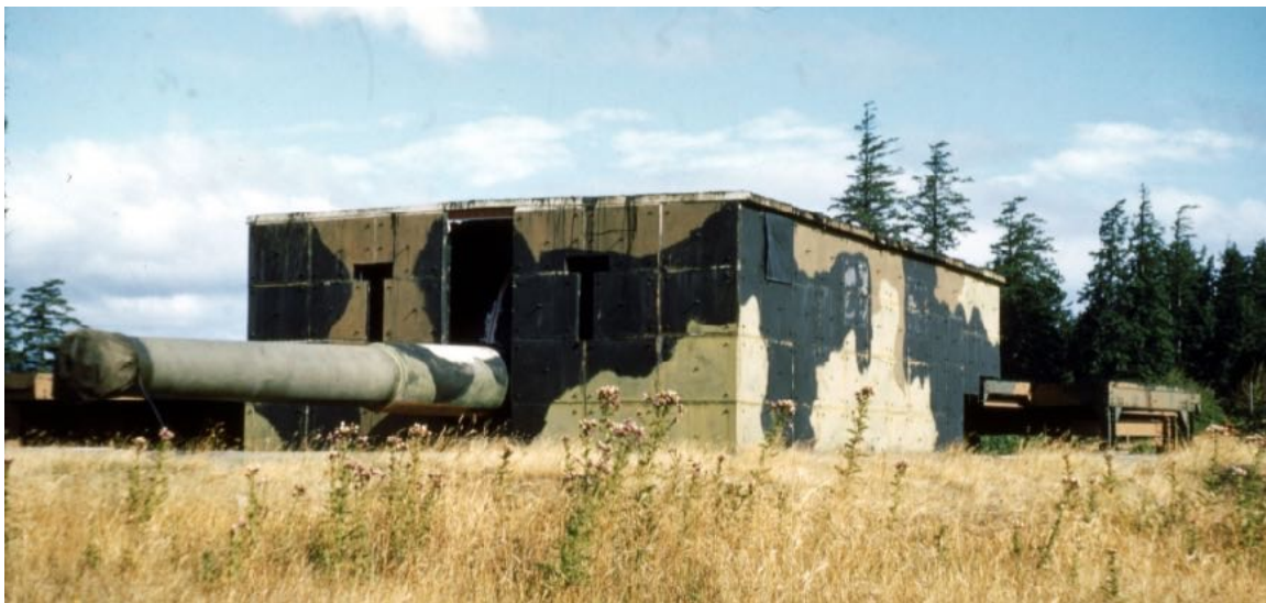
A rare colour photo of a C Mk 6A gun mounting at Albert Head after the Second World War. The slabs from the "plastic armour" can be seen clearly. 15 Field Regiment Archives.
