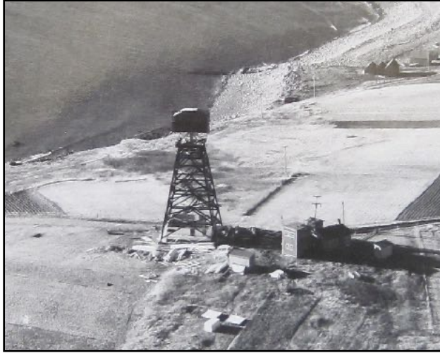
The CD radar site at Osborne Head. Devils Battery Fort Record Book.
