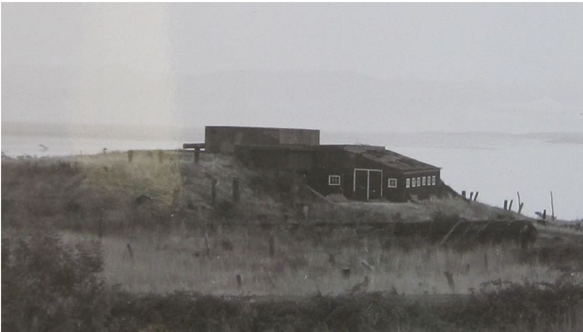
A 9.2-inch gun on a C Mk 6A mounting at Albert Head late in the Second World War. The gun is the box with the pipe on top of the hill and a "farm building" has been built on the rear as camouflage. It also sheltered the rear of the emplacement from the weather. LAC Albert Head Fort Record Book.
