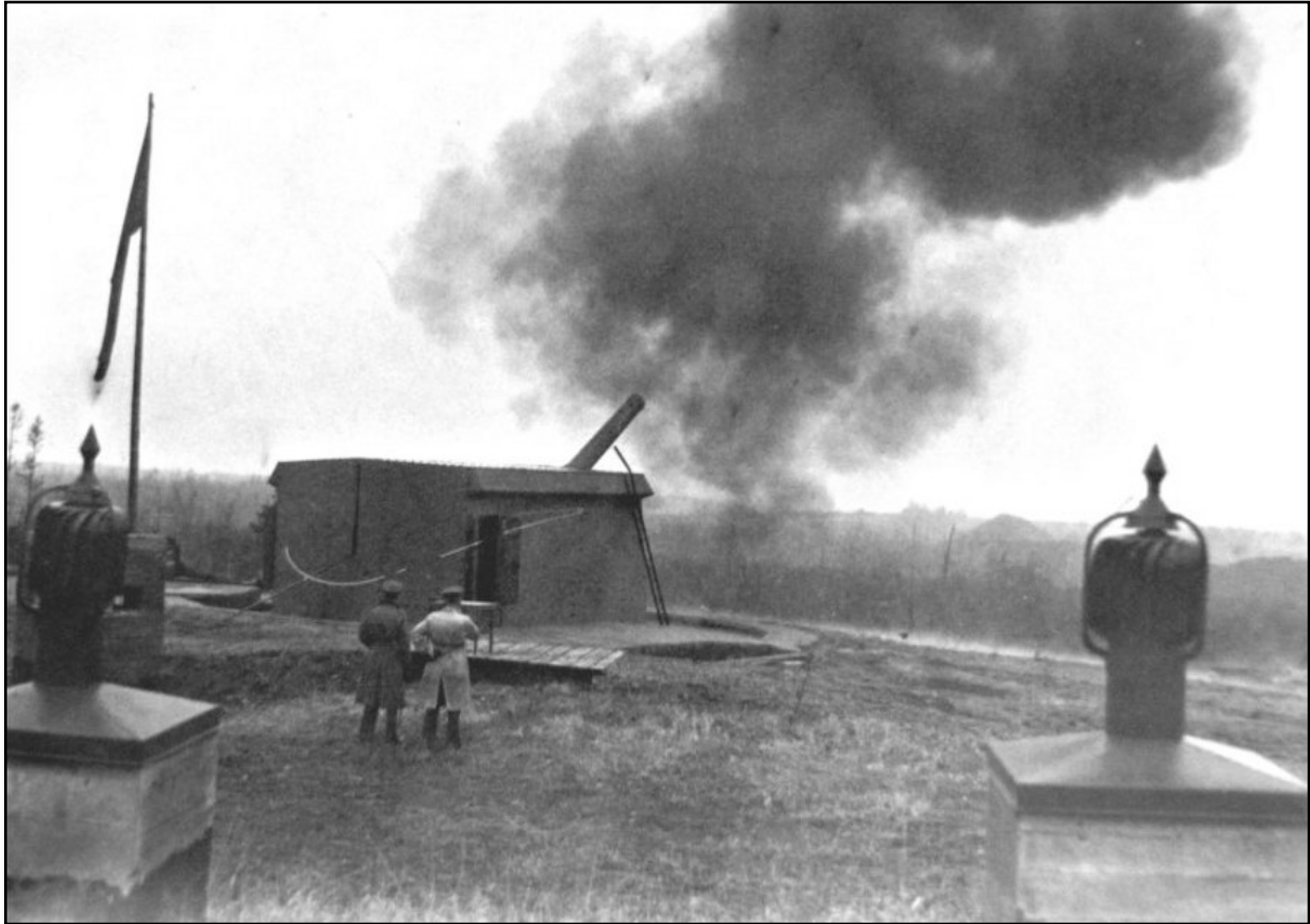
Proof firing a 9.2-inch Mk 15 gun on the Mk 9 Mounting at Oxford Battery after the Second World War. Although the battery was never operational, all three guns were eventually mounted and proof fired. Oxford Battery Fort Record Book.
