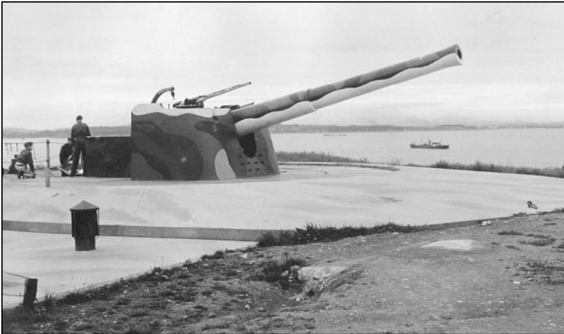
A 9.2-inch Mk 10 gun on Mk 5 Barbette Carriage, probably at Fort McNab in Halifax early in the Second World War. The 6-pounder Hotchkiss sub-calibre gun, and the auxiliary ammunition hoist can be seen above the shield. The men provide a scale for size. LAC 399220.
