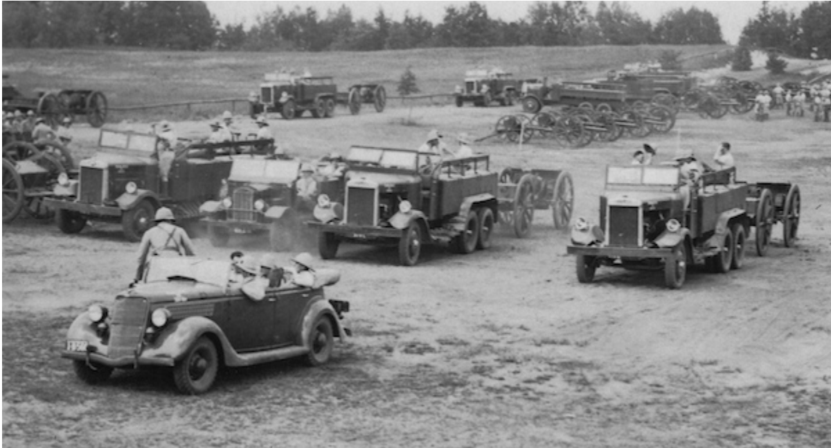
The beginnings of mechanization. 1 RCHA in Petawawa in 1936. Although trucks have replaced horses, the guns are still on their wooden wheels, but with solid rubber tires on the steel rims. This still limited the towing speed of the guns to about that of a horse. Courtesy Jack Holt
