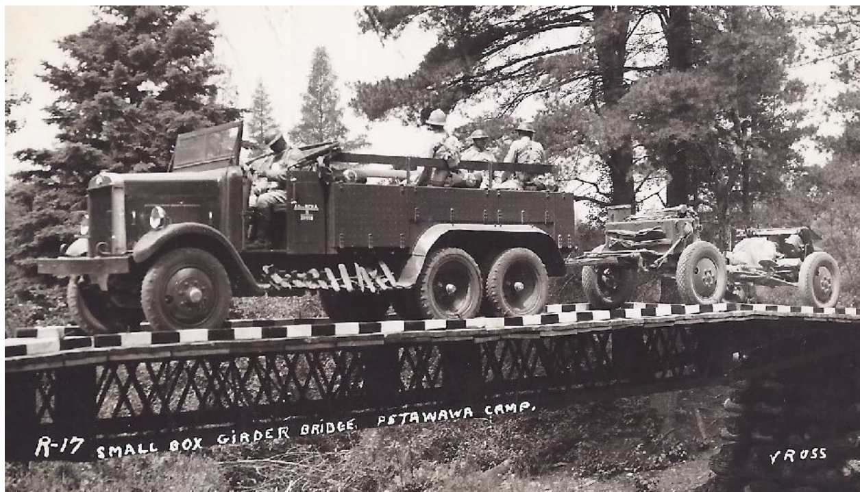
18-pounder participating in trials of the small box girder bridge in Petawawa in late 1930s. The gun and limber have been converted to pneumatic tires. Milart Archives
