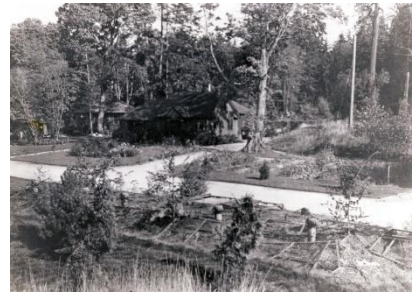
10D – Fort Area. The ventilation shafts to the ammunition magazines can be seen in the foreground with the power house immediately to the rear. The Officers Quarters are to the left. 15FdMuseum
