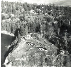
2C– Aerial View. 4 November 1943. This photo shows that the 6” guns have been exchanged with the 4.7” guns from Yorke Island. The overhead, plastic armour structures are complete. Plastic armour was a mixture of bitumen and cement that was originally devised by the Royal Navy as a replacement for concrete slabs which were found to be too brittle. 15FdMuseum
