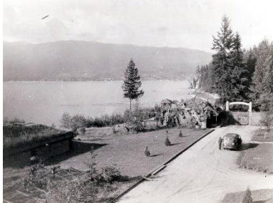
10A – Fort Area. 1945 View looking towards the north gate with No. 2 gun, guardhouse and sentry box visible. 15FDMuseum
