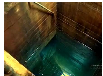
9L – Underground Rooms. 2003. The staircase leading down to the deeper, flooded levels of the ammunition magazine. The Fort Record books states, “During periods of extreme wet weather the magazine floors failed to keep out water seepage until 1-foot drains were cut in the floor and an electric pump was installed.” Could this be the result of removing the pump in 1945? 15FDMuseum.
