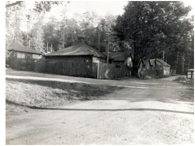
12B – Camp Area. Looking South. Navy Degaussing station in the corner with Salvation Army Hut to the left and 3 Other Ranks Quarters with Guard House to the right. 15FdMuseum
