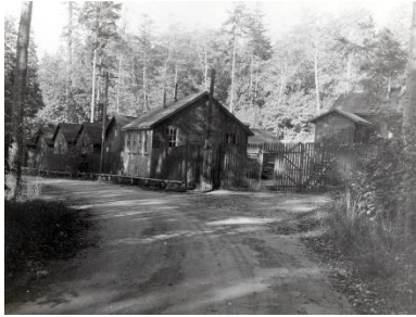
12A – Camp Area. Looking North. Guard House with 3 Other Ranks Quarters behind. 15FdMuseum
