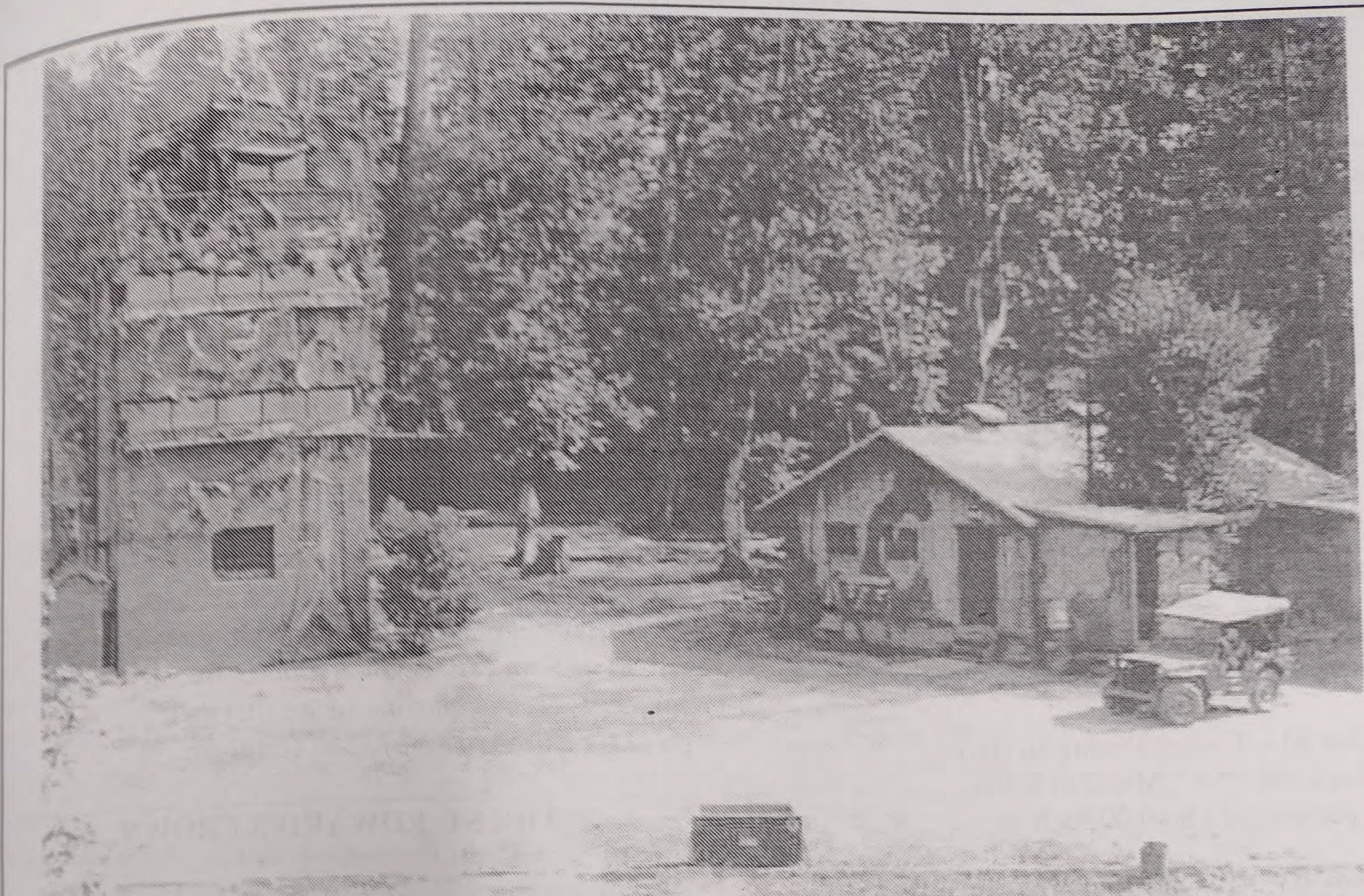
BOP with ELO building to the right. The CP is behind the first row of windows, the op behind the second. The top level is the Signals Hut.
