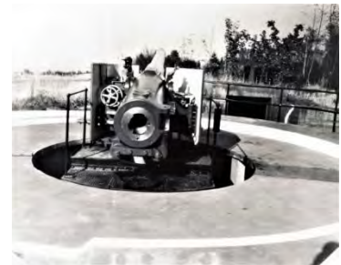
3C – 6 inch Mark VII B.L. Guns on Mk. 2 Mountings. Permanent installation. 15FDMuseum000.15.11B
