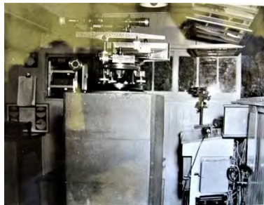
5E – Battery Observation Post. Searchlight D.E.C. control instruments used to control direction of #9 and #10 searchlights. Fort Record Book
