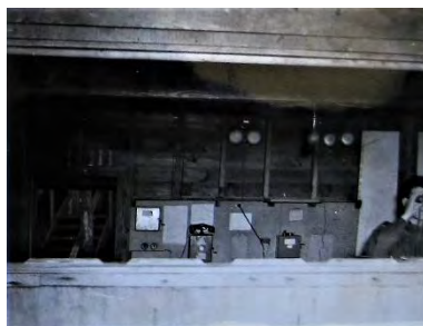
5F - Battery Observation Post. Interior of original, temporary BOP. Fort Record Book
