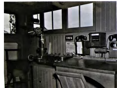
5E – Battery Observation Post. Searchlight D.E.C. control instruments used to control direction of #9 and #10 searchlights. Fort Record Book
