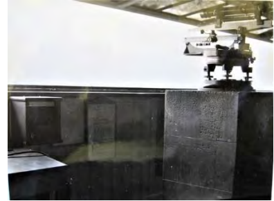
5C – Battery Observation Post. The new BOP was equipped with a Depression Range Finder (DRF) Mark V and Magslip Transmission. Photo shows the DRF. Fort Record Book
