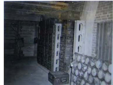
6C – Ammunition Magazine. 1974. The remains of the ammunition hoist in the shell magazine. 15FdMuseum
