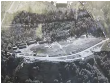
2B – Aerial View. A good view of the camp layout. It appears that the concrete work on the permanent emplacements has just recently been completed as no backfill has taken place yet.
