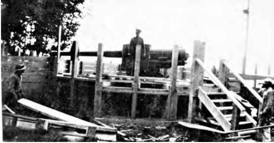
3A – 6 inch Mark VII B.L. Guns on Mk. 2 Mountings. Temporary installation September 1939. 15FDMuseum985.13.2
