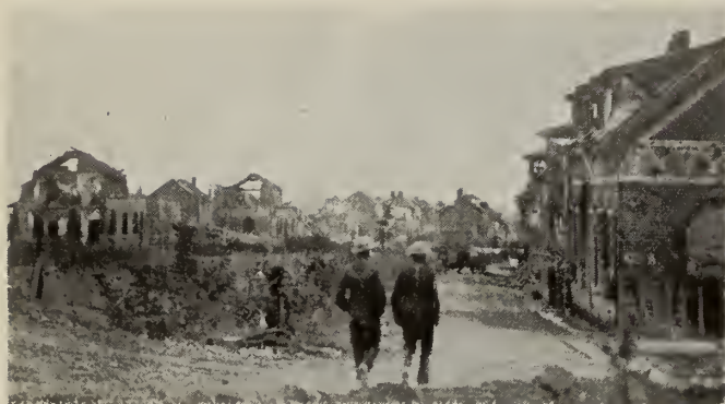
In the cellars of such houses as these soldiers made their homes.
