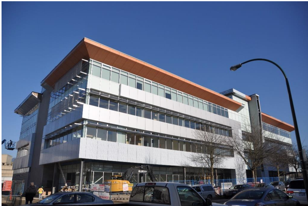
The new Jericho Replacement Building. DND/CAF organizations will be relocating from Jericho Garrison to the JRB later in the year. Photo by Capt Chris Poulton, 39 CBG Public Affairs
