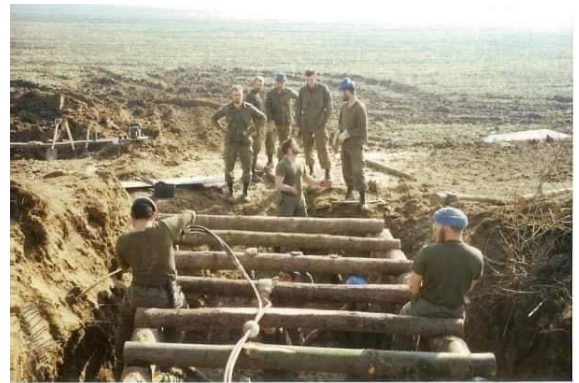
Canadian pioneers build a bunker in Croatia in 1992. Private collection of Maj Brian Hynes
