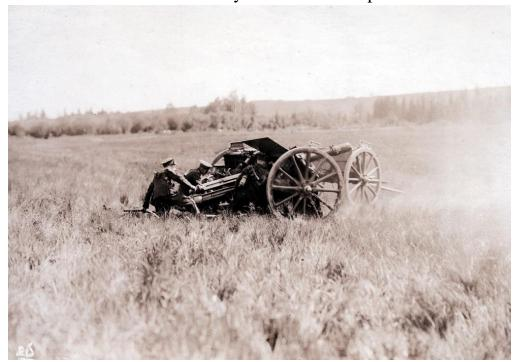
being fired at Sarcee. What looks like a "muzzle cover" is actually a canvas cover to protect the oil and nitrogen gas valves in the large recuperator cylinder, which was mounted above the tube. You can see the muzzle itself just to the right of the vertical spoke in the right wheel. The leather ammunition pouches, worn by the gunners here, were eventually replaced by webbing pouches, a process actually under way in 1914, although the Reserves didn't
