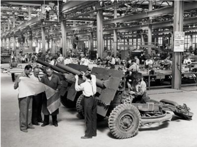
Workmen constructing 25-pounder guns in Sorel, 1941. Photo by Nicholas Morant. National Film Board of Canada / National Archives of Canada, PA-174507.
